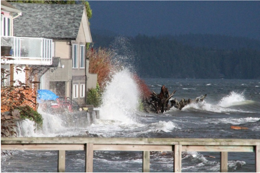
Looking north past Armours Beach to wave impact on shoreline homes
